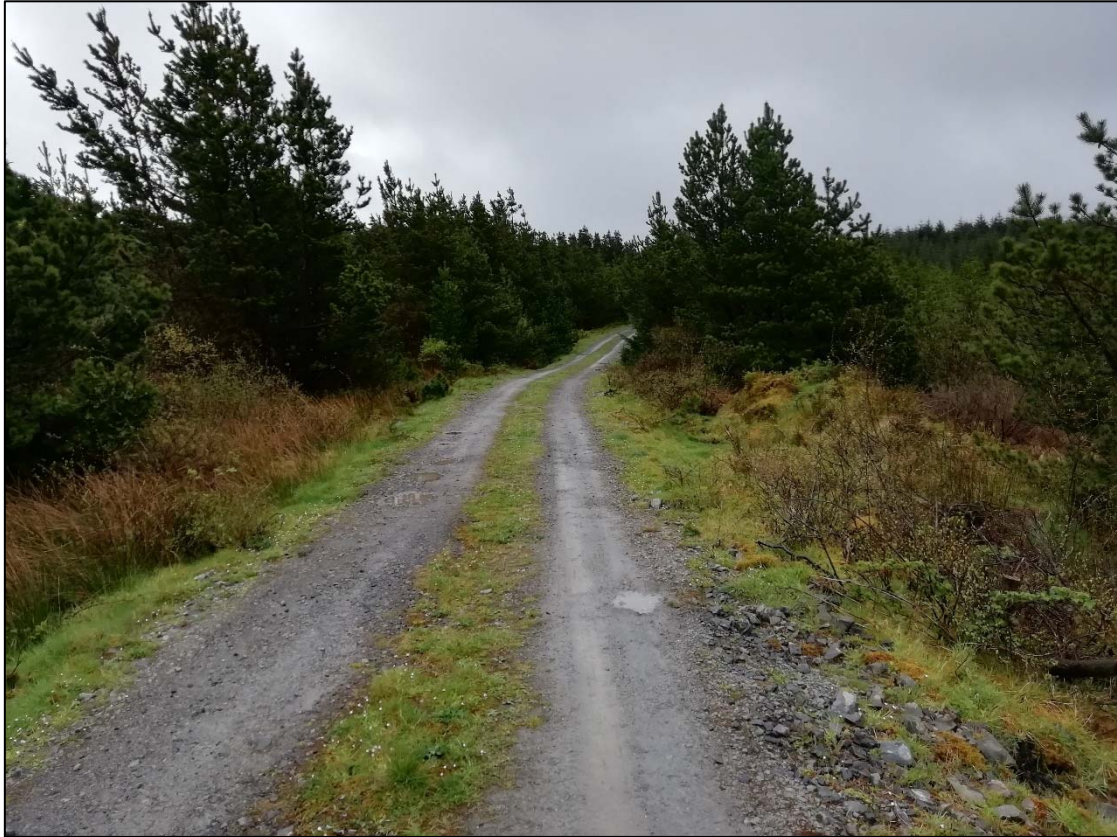
Plate 6-9 Example of existing unbound forestry tracks categorised as Spoil and bare ground (ED2)
